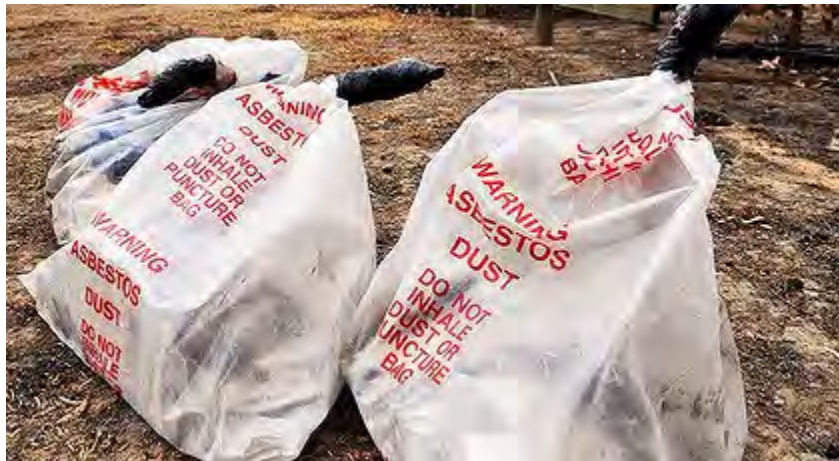
Figure 8d 47 : Example of airtight, labelled double bags packed with ACM
